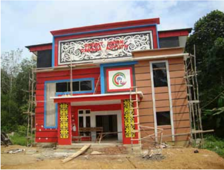
The construction of the office of Canaga Antunt Credit Union. Photo credit: ID
