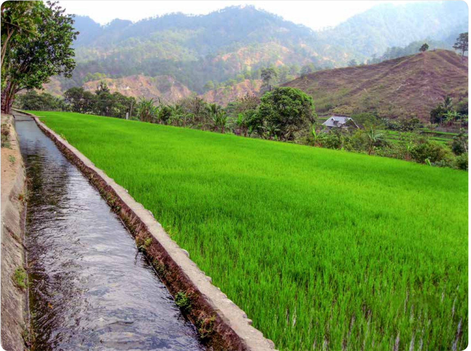
Water from creeks is channelled to a power canal, then to a penstock (right).
