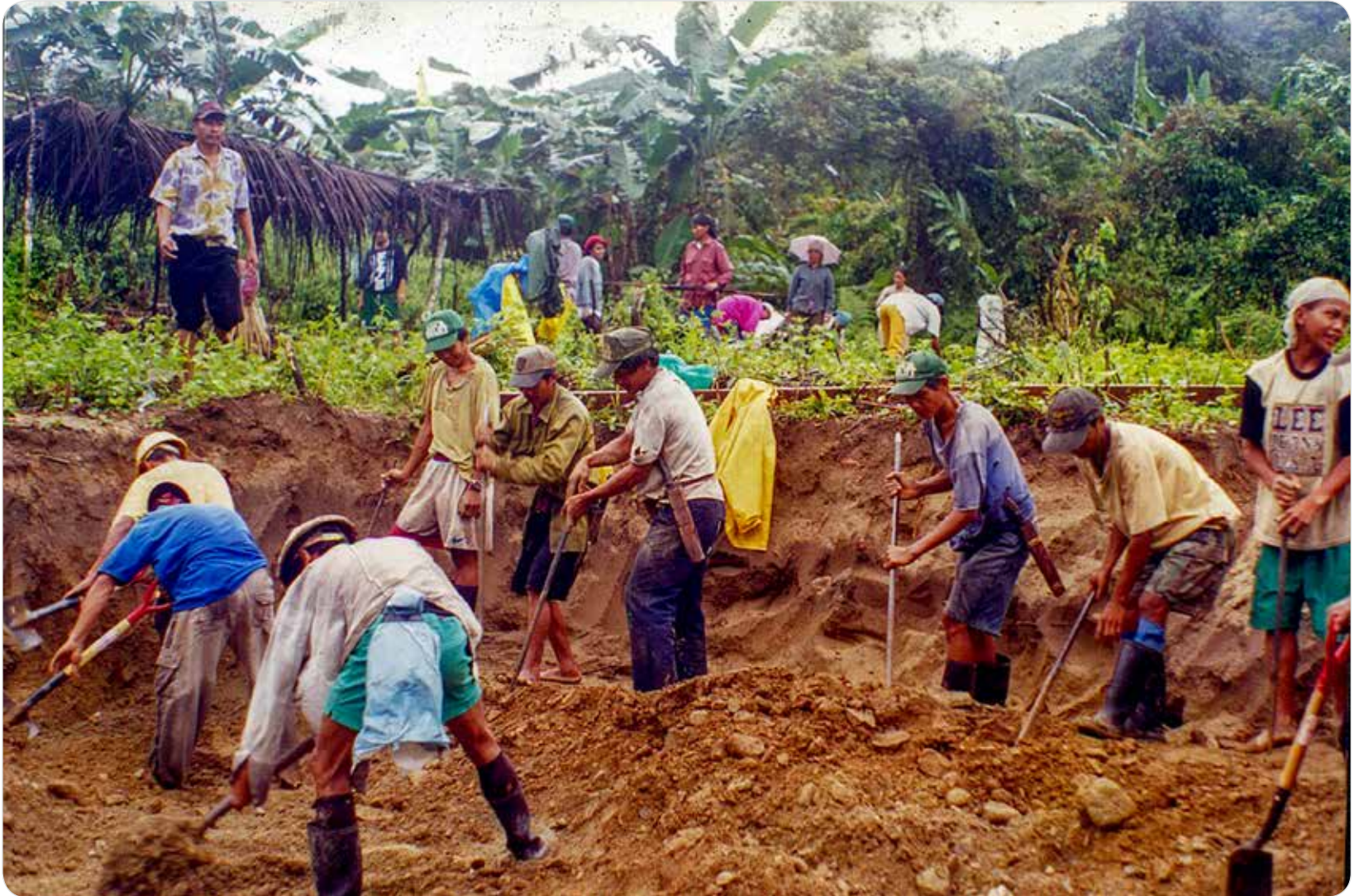
Cooperative labor in construction of the powerhouse.
