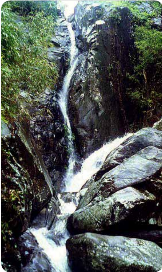
The 50-meter head from the Caguyen Falls in Baay-Licuan in Abra provides 17.5 kW of power for the microhydro of Sitio Caguyen.
