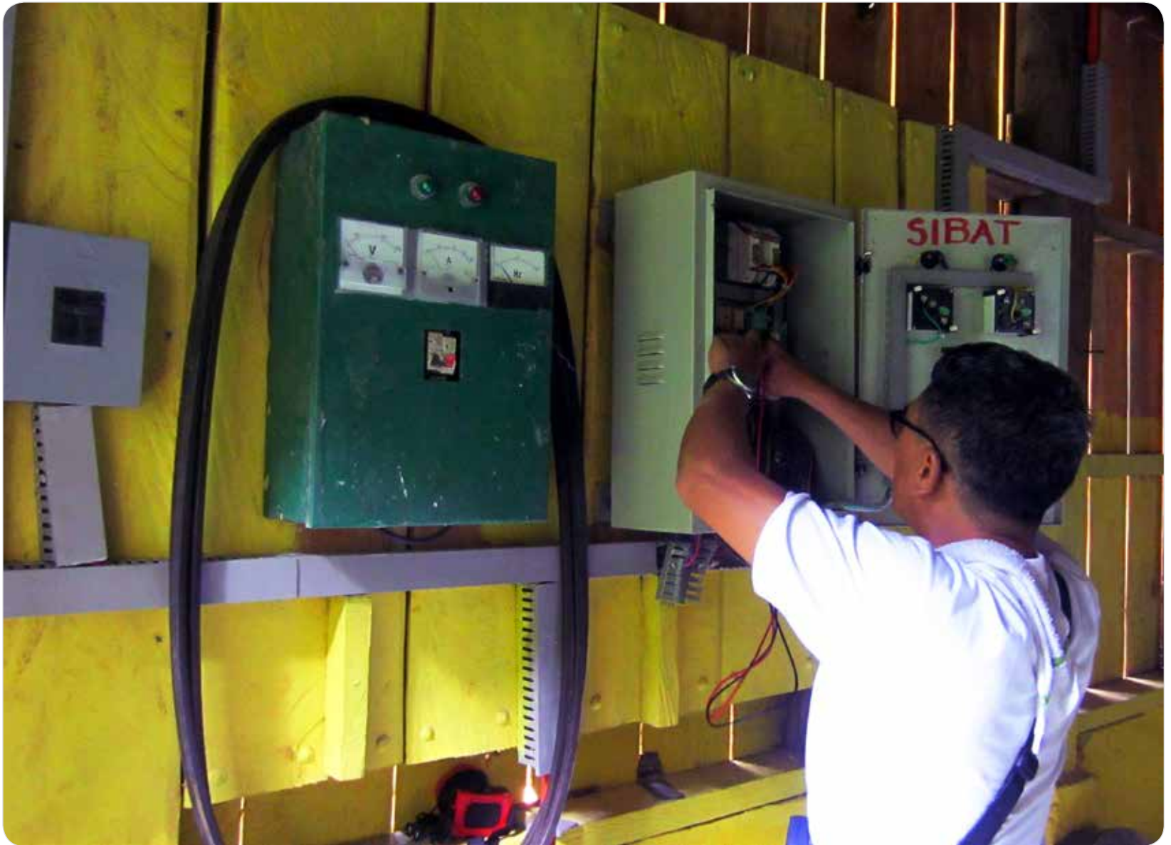
The Electronic Load Control enables 24-hour operation.
