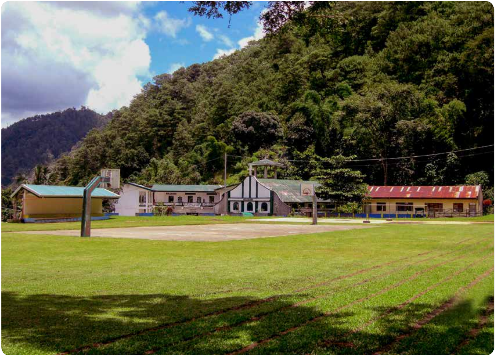
A 20-kW microhydro provides electricity for the 154 households, schoolhouse, church and parish of the indigenous Banao community in Balbalasang, Balbalan, Kalinga.
