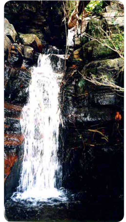
The 50-meter head of Desay Waterfalls forming the Desay Creek at the foot of Mt. Alibanua, provides 5 to 21 kW of power for the run-of-river MHP for the community of Bagong Bayan, Roxas, Northern Palawan.
