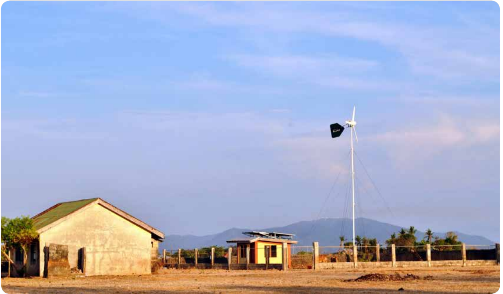
Wind turbine supply built in Sitio Buli, Cabra Island, Municipality of Lubang, Occidental Mindoro.
