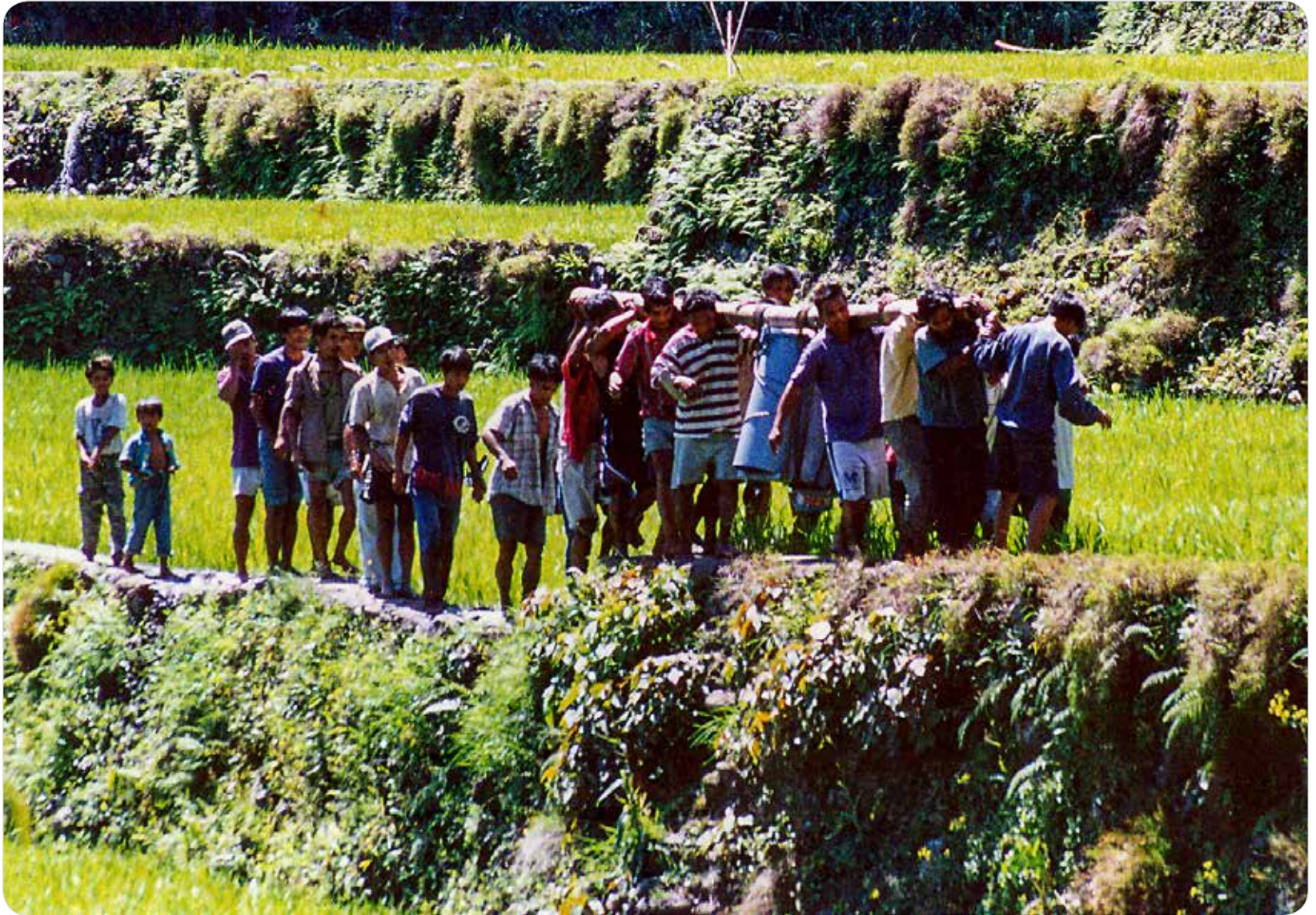
Traditional cooperative labor is practiced in doing the many tasks of building the microhydro.
