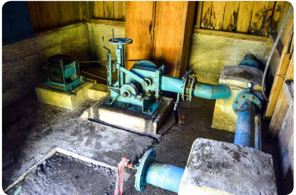
The crossflow turbines of Katablangan microhydro (left) and Bubog microhydro (below).
