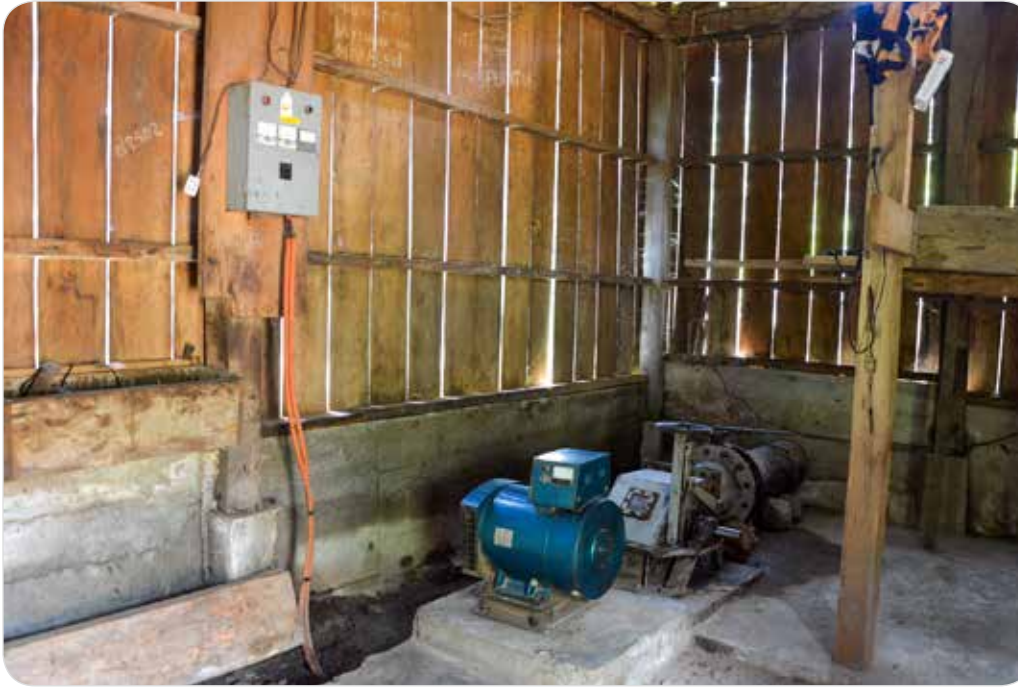
The crossflow turbines of Katablangan microhydro (left) and Bubog microhydro (below).
