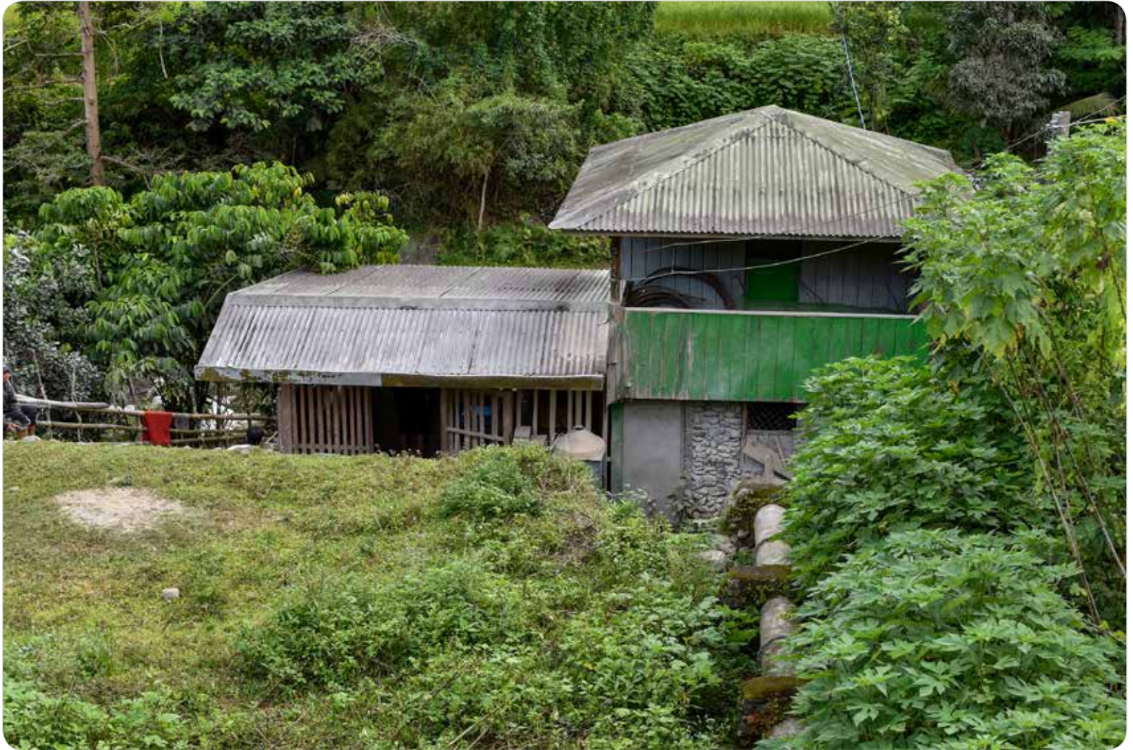
The penstock runs into the powerhouse which houses the electromechanical heart of the microhydro, the turbine.
