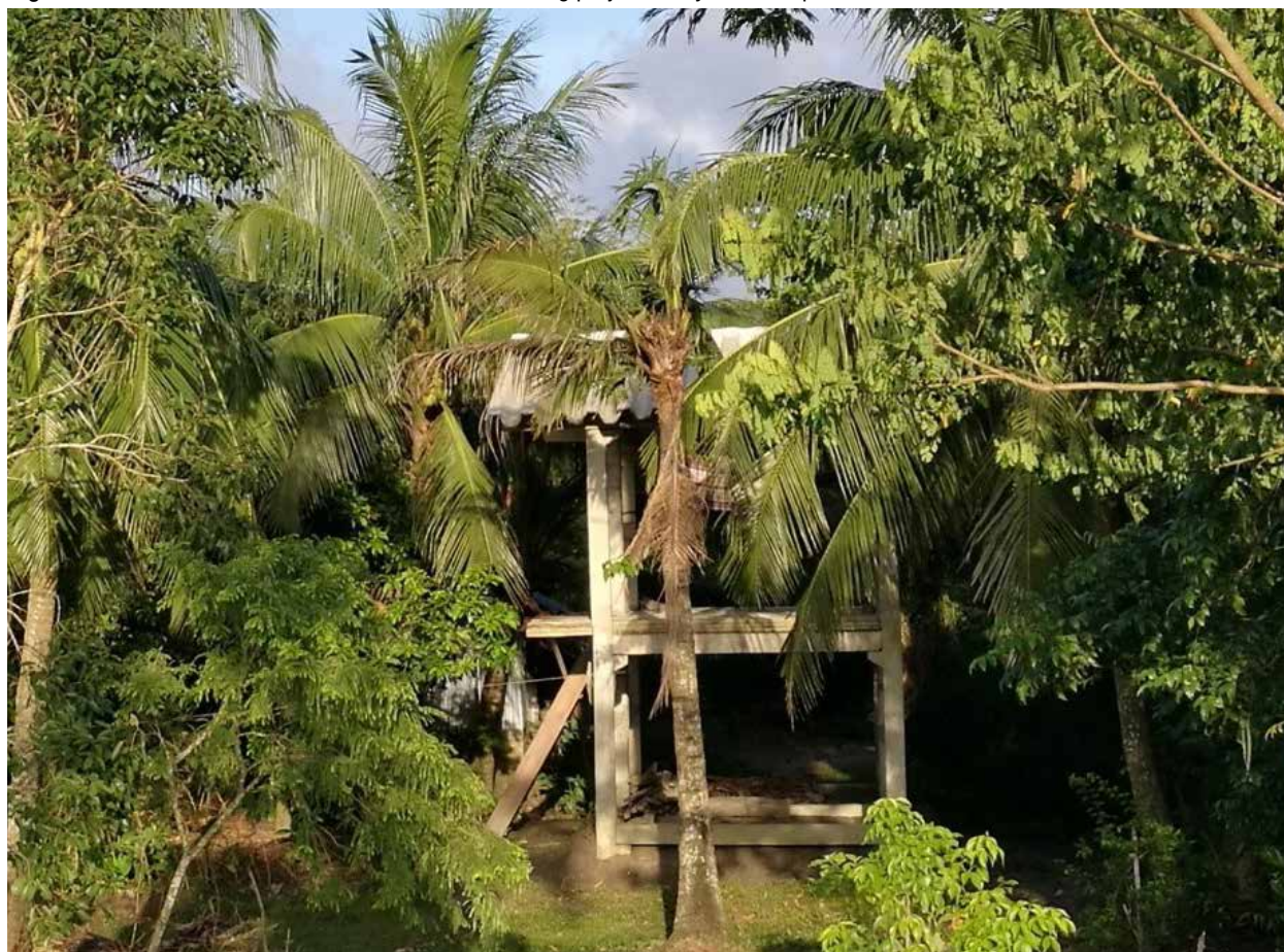
Figure 3. Climate resilient house built under the housing project Asroyon Prakalpa-2.
