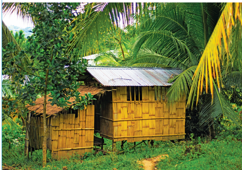
Most houses in the Lambangian community in the Philippines are made with light materials like kawayan (bamboo) and cogon grass which are readily available in their ancestral domain. Benuan, Kuya, South Upi, Maguindanao, Philippines
