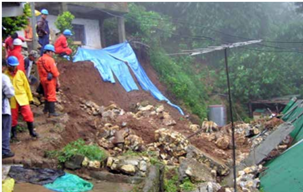
Figure 14. Landslide in Baguio City.
