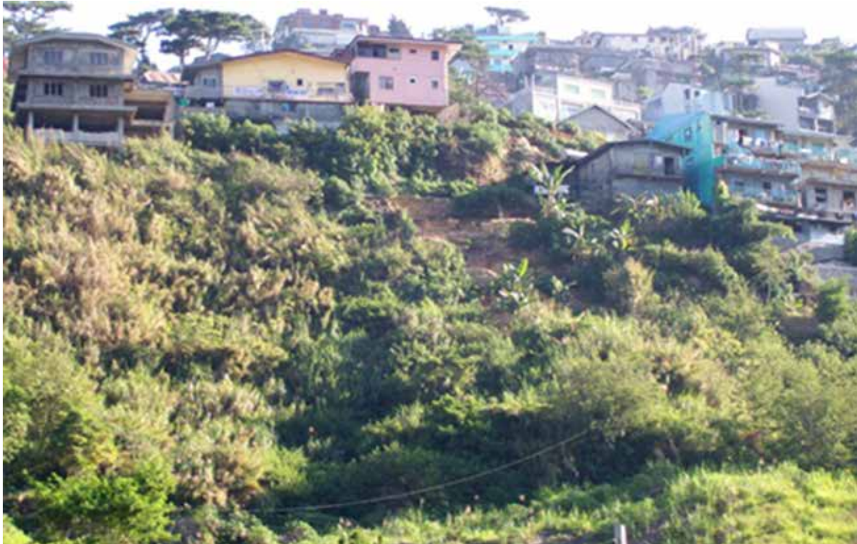
Figure 5. Residences constructed in steep, landslide-prone area.
