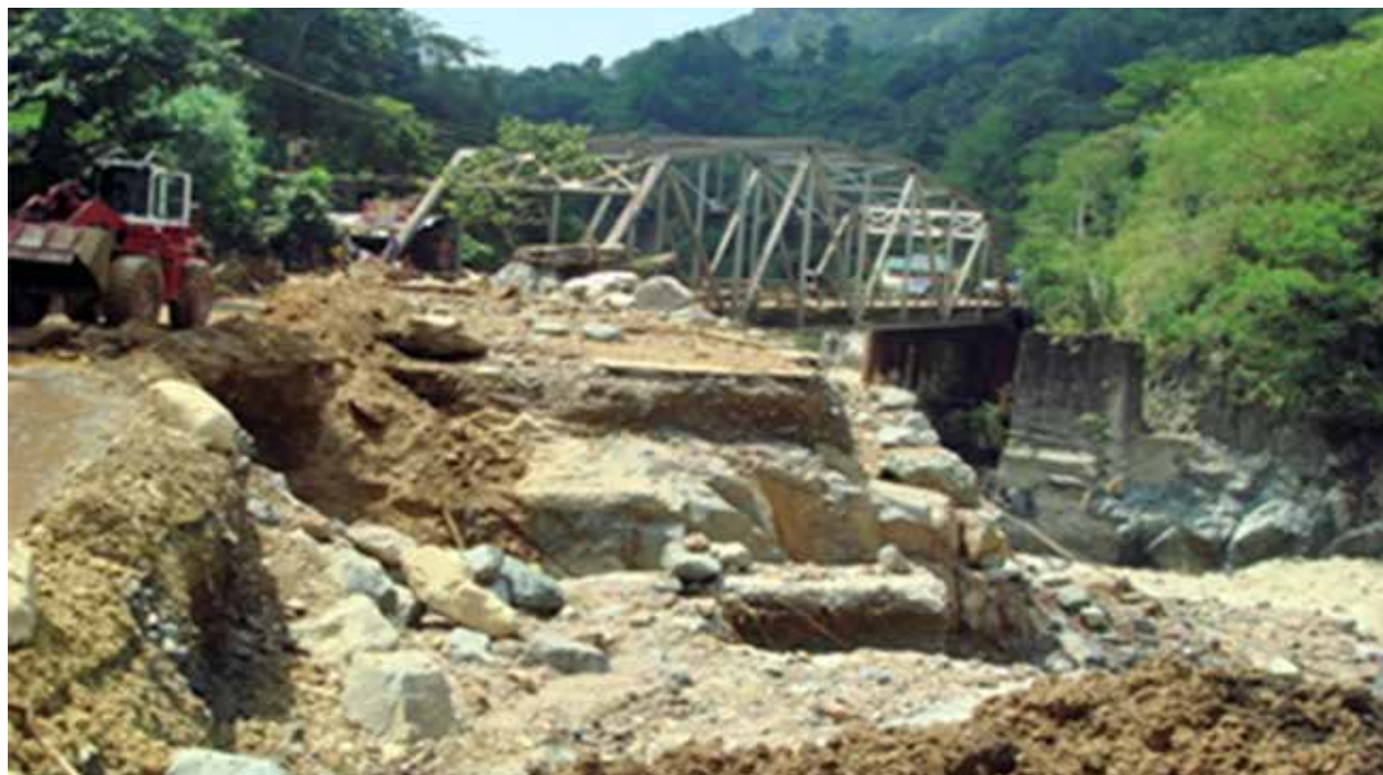
Figure 15. Roadcut along Kennon Road leading to Baguio City
